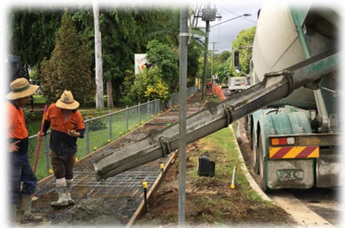
The new 'MRTS36' specification Glass Aggregate product & it's use in construction works.
